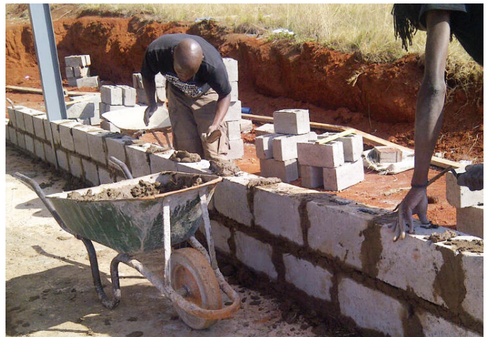
Local brick-makers building the walls of the library
