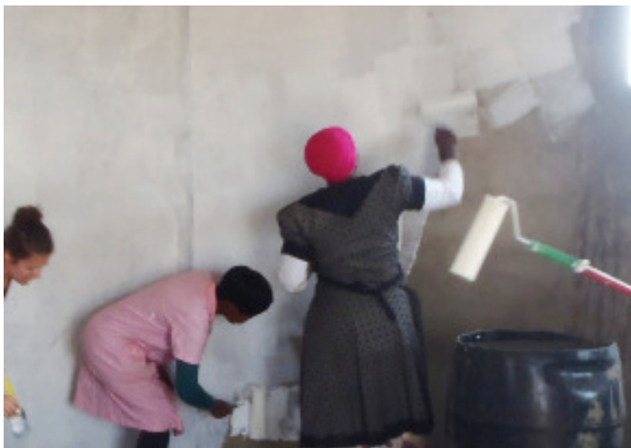
MSP staff and volunteers painting the inside walls
